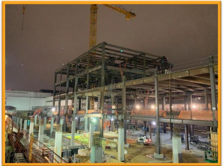
*Above: Steel erection continues on the future Head House building between Terminals 2 & 3*
