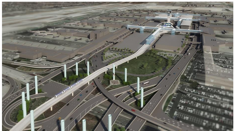
The LAX Train (Automated People Mover) will be above grade, allowing the system to avoid airport roadways, and will connect passengers to airport terminals from convenient locations outside the airport's Central Terminal Area.
