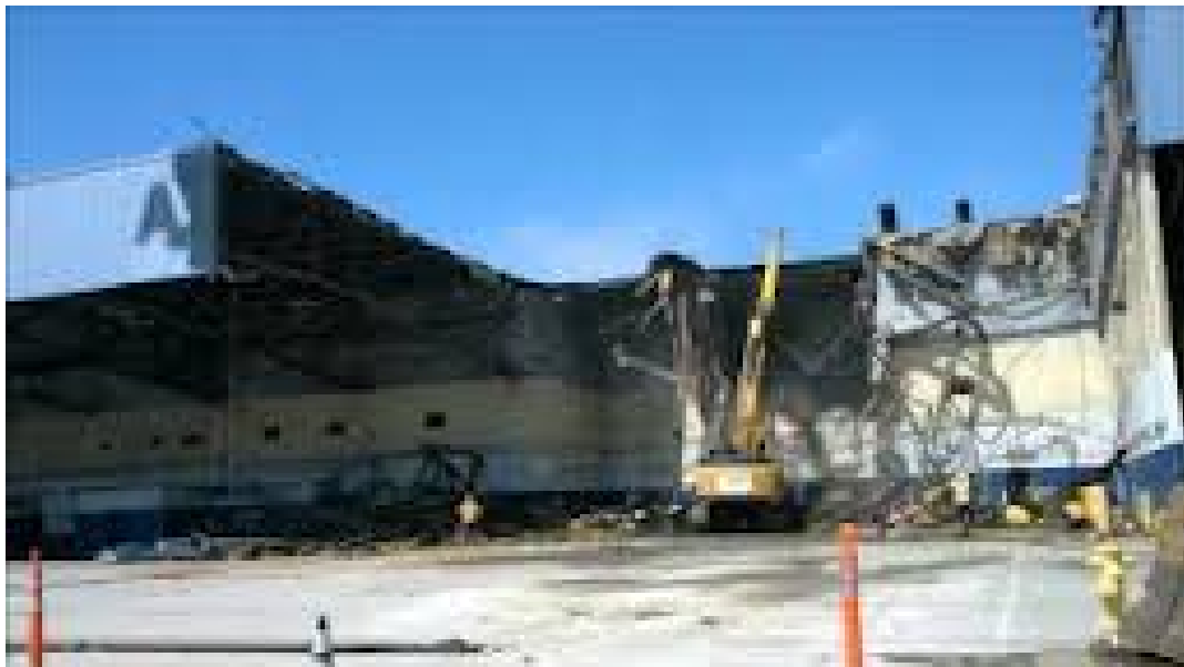
Figure 1.2.2-1: American Airlines Hangar Demolition in Progress – August 13, 2012
