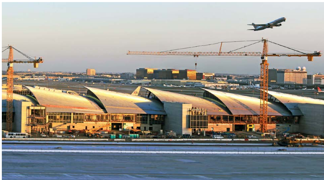
Figure 1.2.2-2: Tom Bradley International Terminal Project Under Construction at LAX
